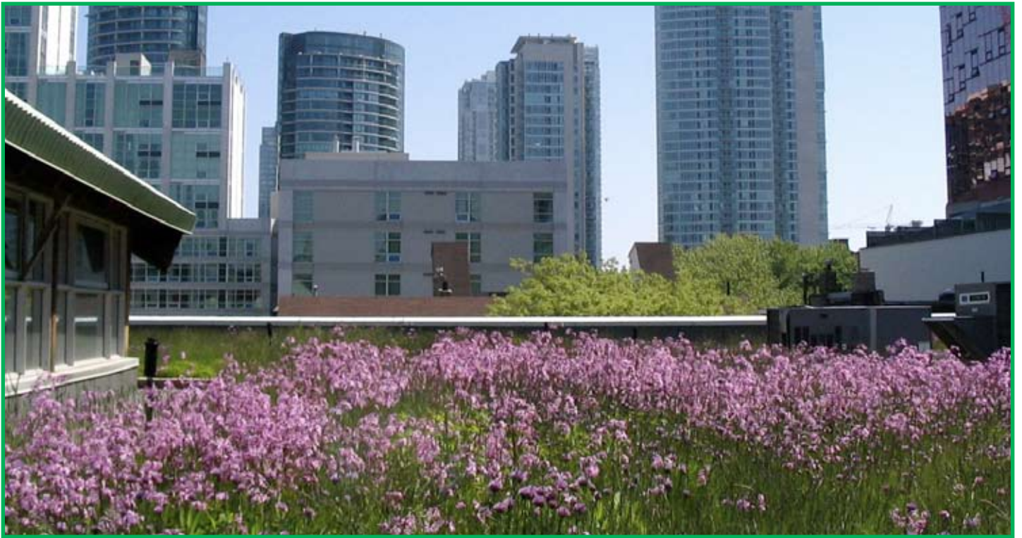
Green roof at Mountain Equipment Coop, Toronto, Canada – a sight which should be much more common in the UK
